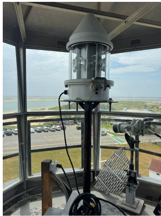
The team seats the new lighting system on its post, the new light ready to shine Matt Provost photos
