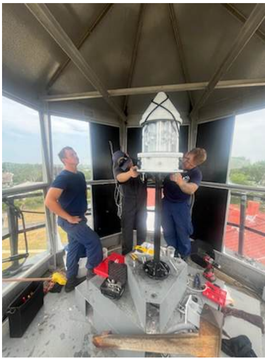
The team seats the new lighting system on its post, the new light ready to shine Matt Provost photos
