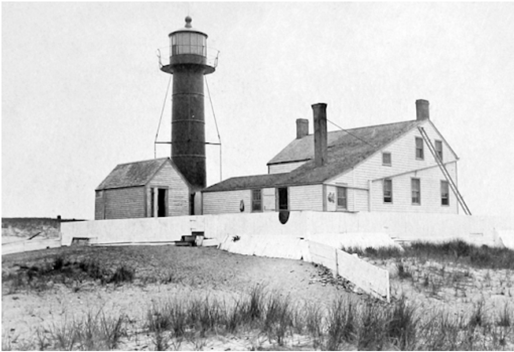
Circa 1890: tower upgrades included red paint, guy wires, and a sand fence. Note the gutters used to channel rain water from the roof of the house to the basement cisterns.
