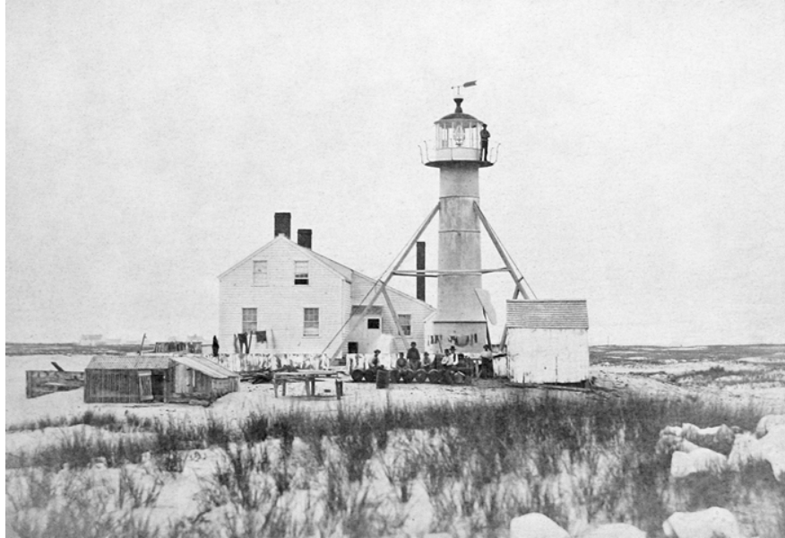
Monomoy Lighthouse circa 1850: both the tower and dwelling were painted white and bracing helped stabilize the tower -courtesy Chatham Historical Society
