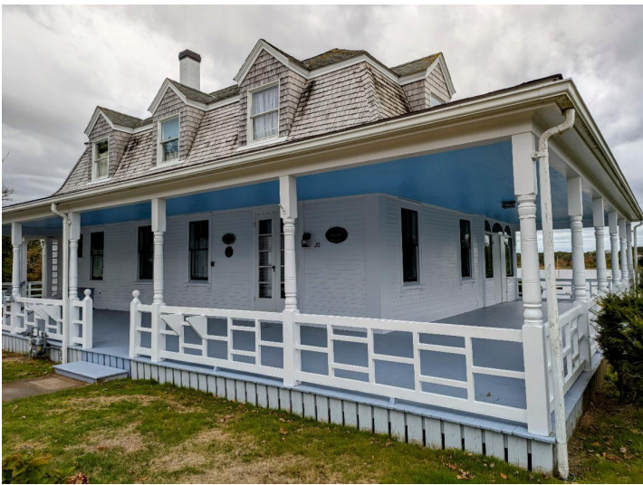
Porches freshly painted. photo © EJH 2024
