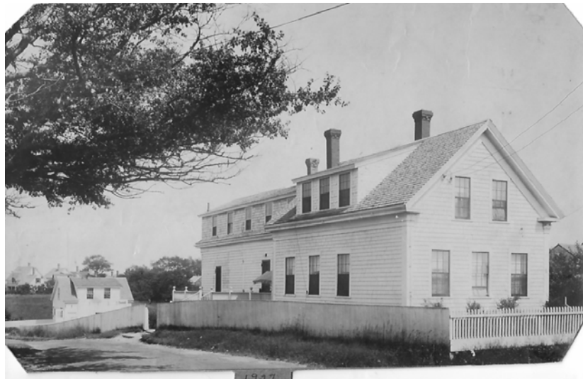
North side of the house including the garage, 1927. Courtesy the author.
