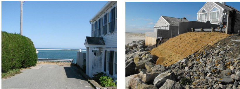
Water Street Town Landing, a work in progress
