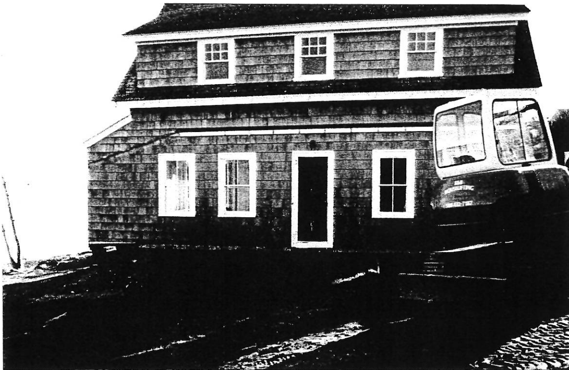
100 Main Street Ready for Renovation
